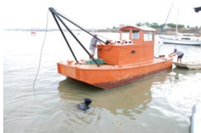
Diver attaching cable to adjust mooring buoys The water is indeed brown and the diver only wears a mack and snorkel
