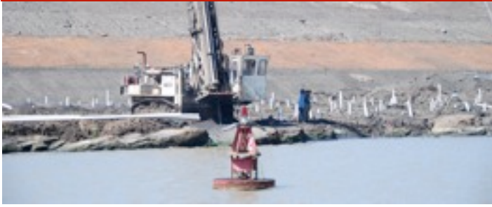
Left : Widening the canal is a challenge...
